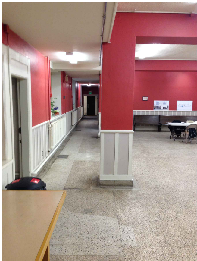
IMAGE 2/A1.01 EXISTING COLUMN COATING
